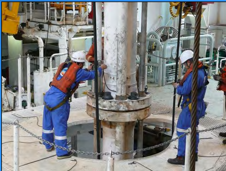
Installation of RALS (Riser Angle Logging System)
