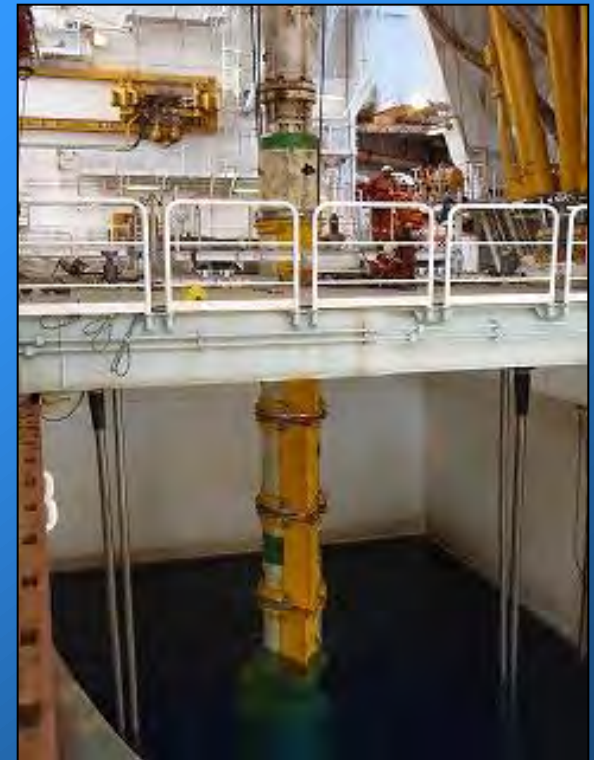
Installation of Riser Fairings
